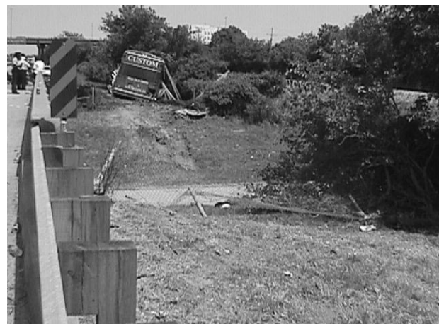
Figure 1: A photograph showing the final rest position of the accident bus after it impacted the embankment above the golf cart underpass.
