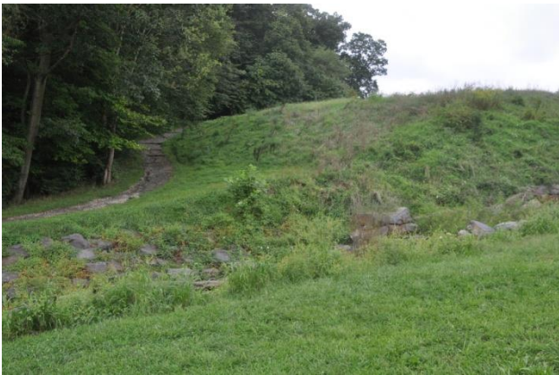
Figure 2. Slope where incident occurred.
